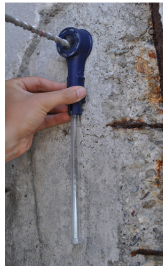
Drilling phase with powder collection for carbonation test
